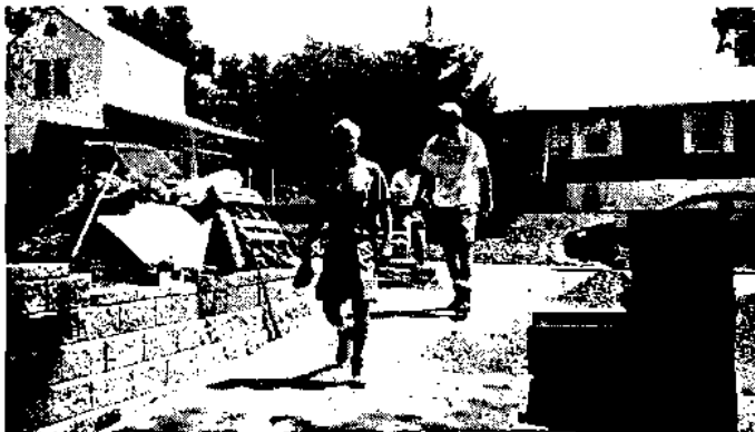
We will get this water problem solved and build these driveway walls
