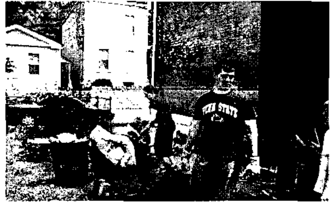
I H M youth remove old carpet & prepare site for the blitz crew at 213 Bush Street.
